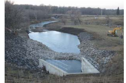
Looking downstream from outlet structure
