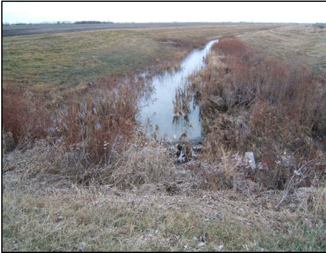
Area of sediment and willows to be cleaned out of Burnham Creek
