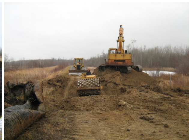
Repair of Dike after Removal of Structure
