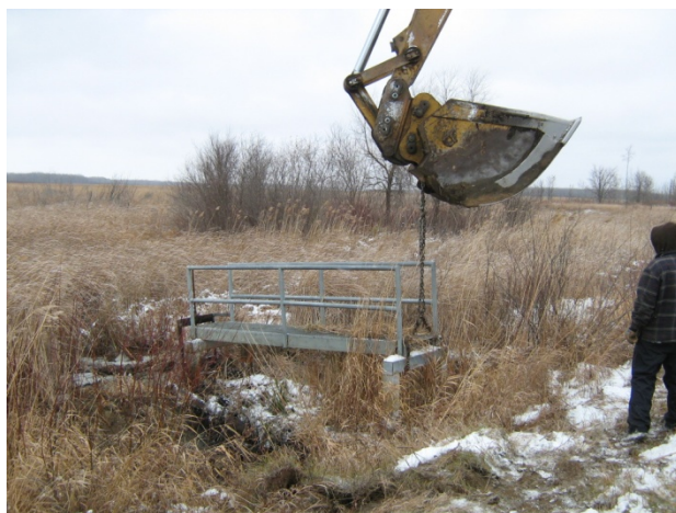
Removal of Walkway and Gate Structure
