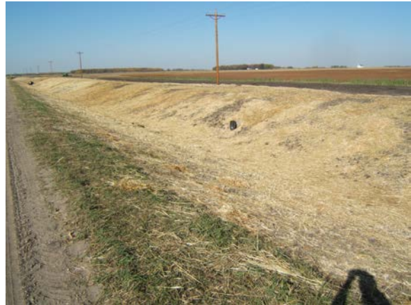
Looking west at Station 24+33
