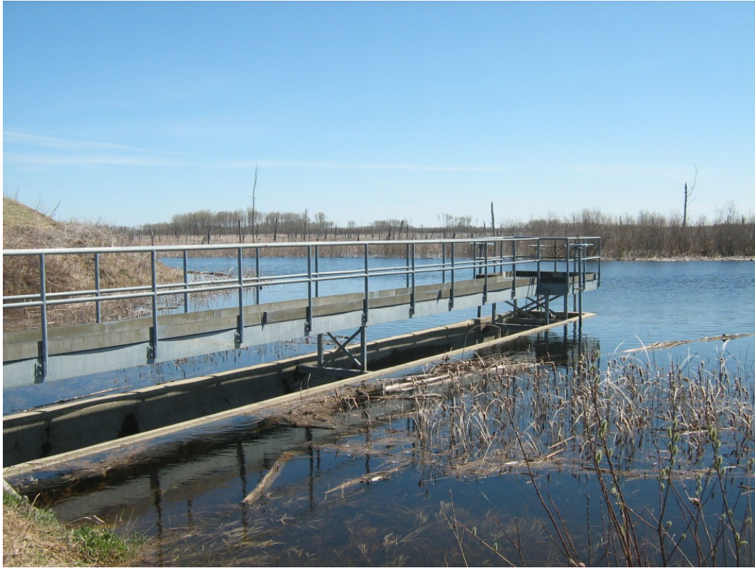
North Pool - Gated Principal Outlet Structure
