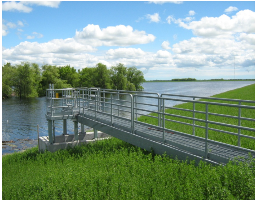
Principal Outlet Structure
