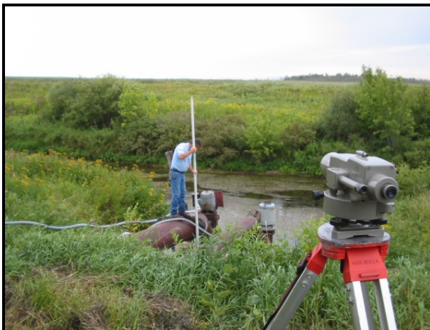
Surveying water lift from river to pump
