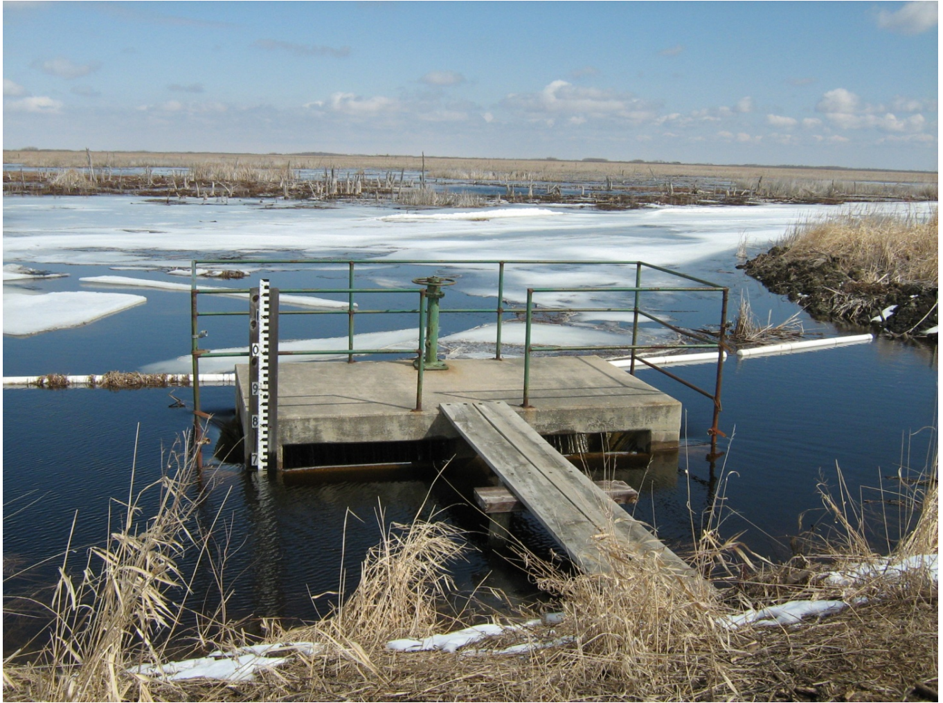
Gated Outlet Structure
