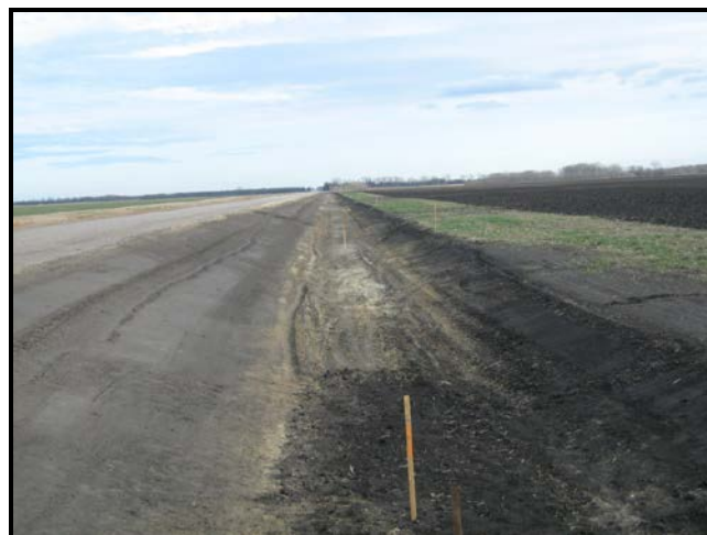
Example of well done excavation
