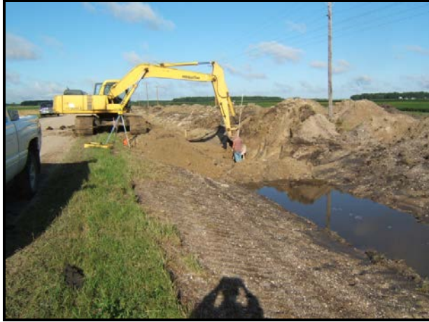
Preparing bed to install a field crossing
