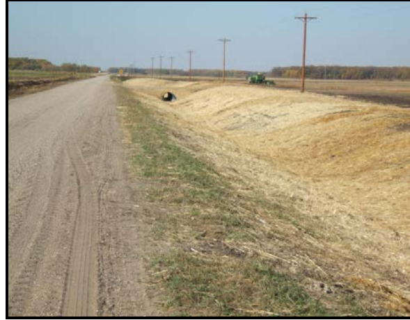
Ditch work completed and seeded and mulched
