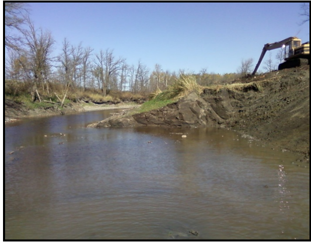
Cleaning sediment bar from Ditch 83
