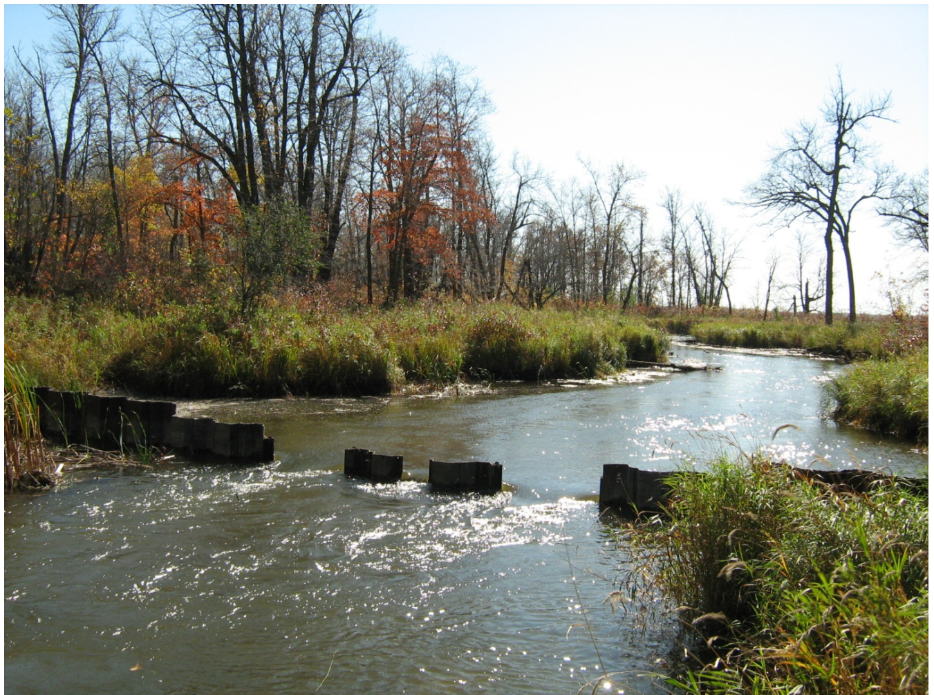
Typical Fall Drawdown with Stoplogs Removed
