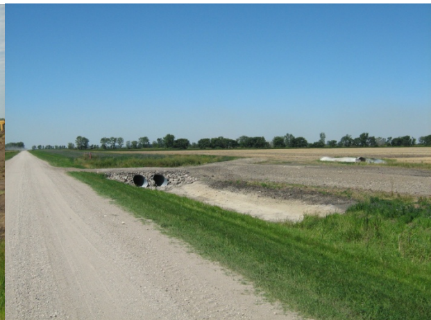
Field Entrance Site and Berm
