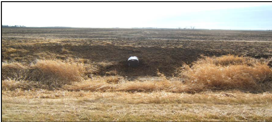
One of several new Side Water Inlet pipes installed in RLWD 3
