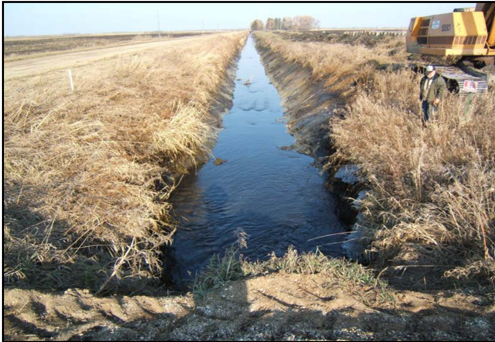
JD 72 cleaned and flowing, Rock rip-rap to be added
