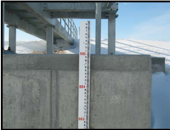
Typical staff gage at structure
