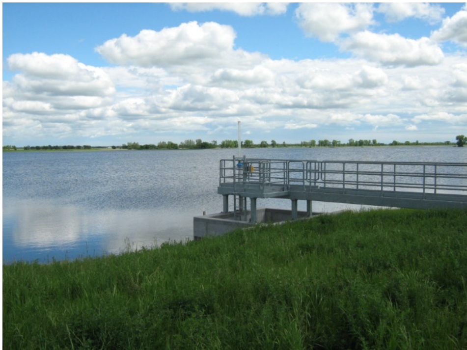
Principal Outlet Structure
