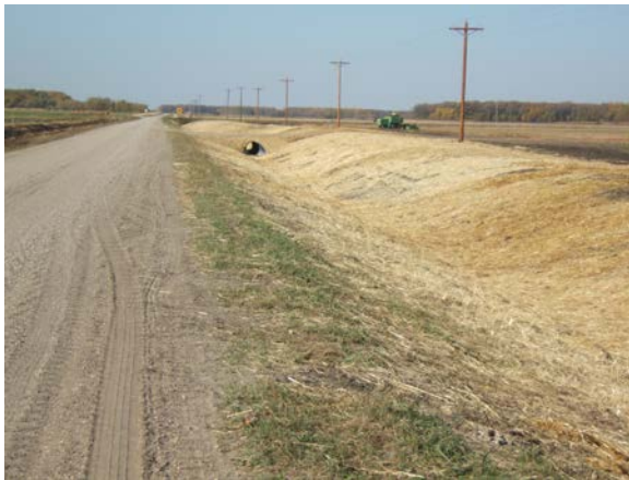
Looking west at Station 14+00
