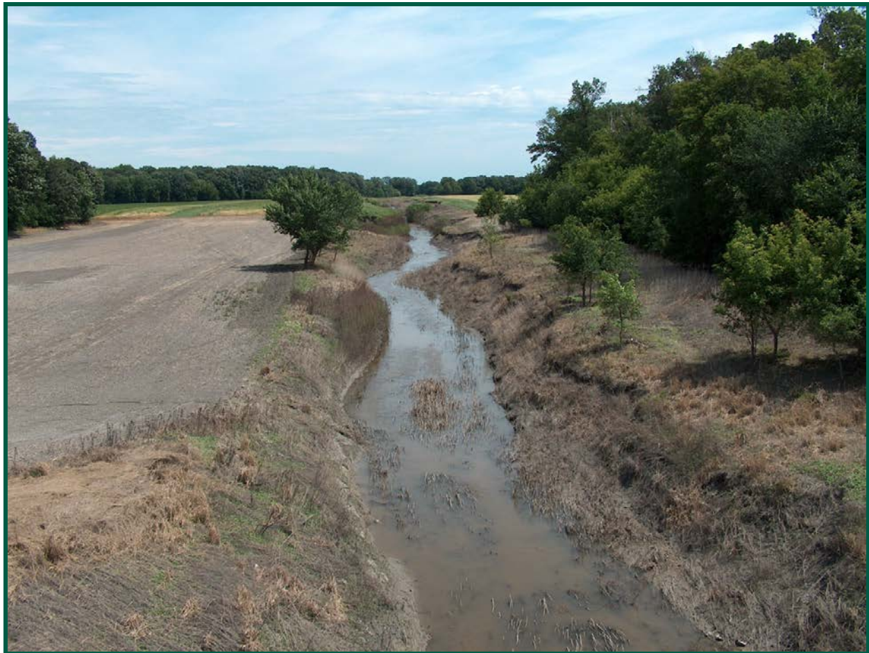
Looking east at cut-channel from CSAH #64
