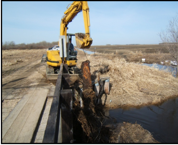
Removing log jam from the bridge
