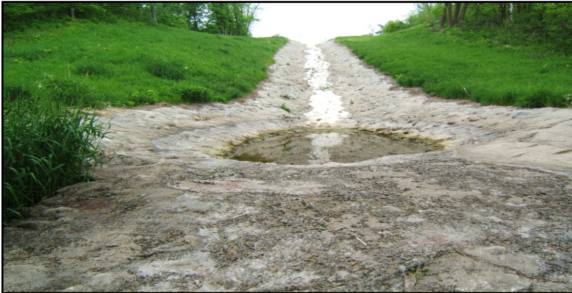
Rock chute at the outlet of RLWD Ditch #10
