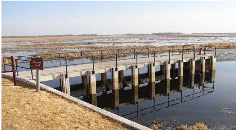
Stoplog Outlet Structure
