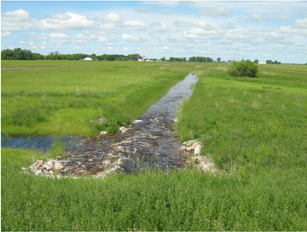
Principal Outlet Structure – looking west
