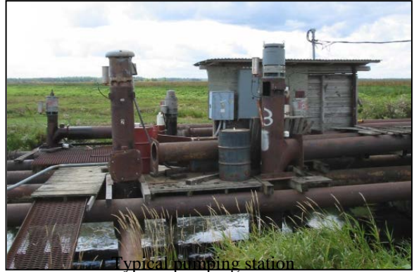
Typical pumping station
