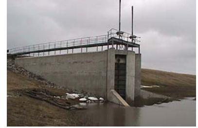
Principal outlet structure hydraulic gate operation
